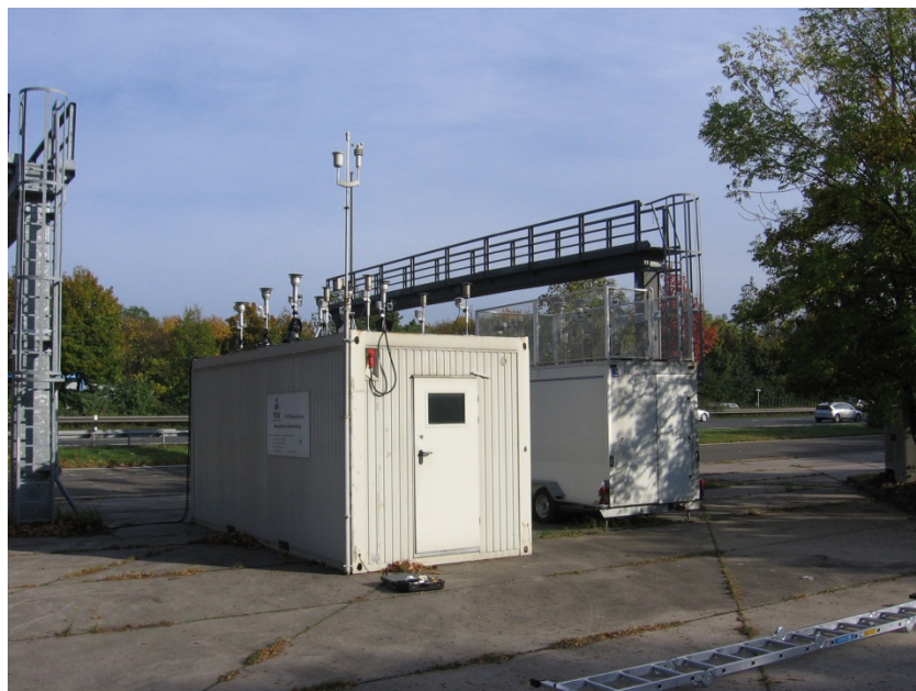
Figure 19: Field test site Bornheim, motorway parking lot
